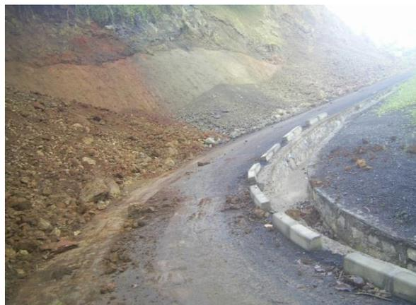
**Figure B.10 Landslide on Moheli, Comoros, induced by moderate earthquake and tropical cyclone Hellen (Source: Mansourou, 2014)**
