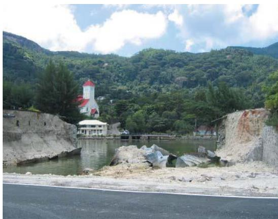
**Figure B.8 The remains of a road swept away by the tsunami (photo taken from repaired section).
