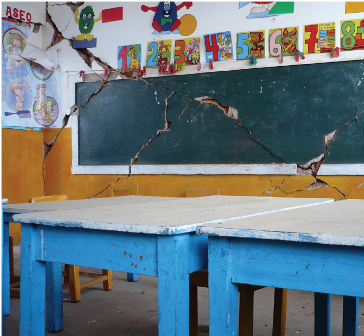
In 2007, the Picaso earthquake in Peru rendered this primary school classroom unsafe for use. Heavily damaged learning facilities must often be torn down. Moderate changes to design and construction can reduce the likelihood of heavy damage and ensure children have access to education, even after disaster strikes. Photographer: Claudio Osorio, INEE
