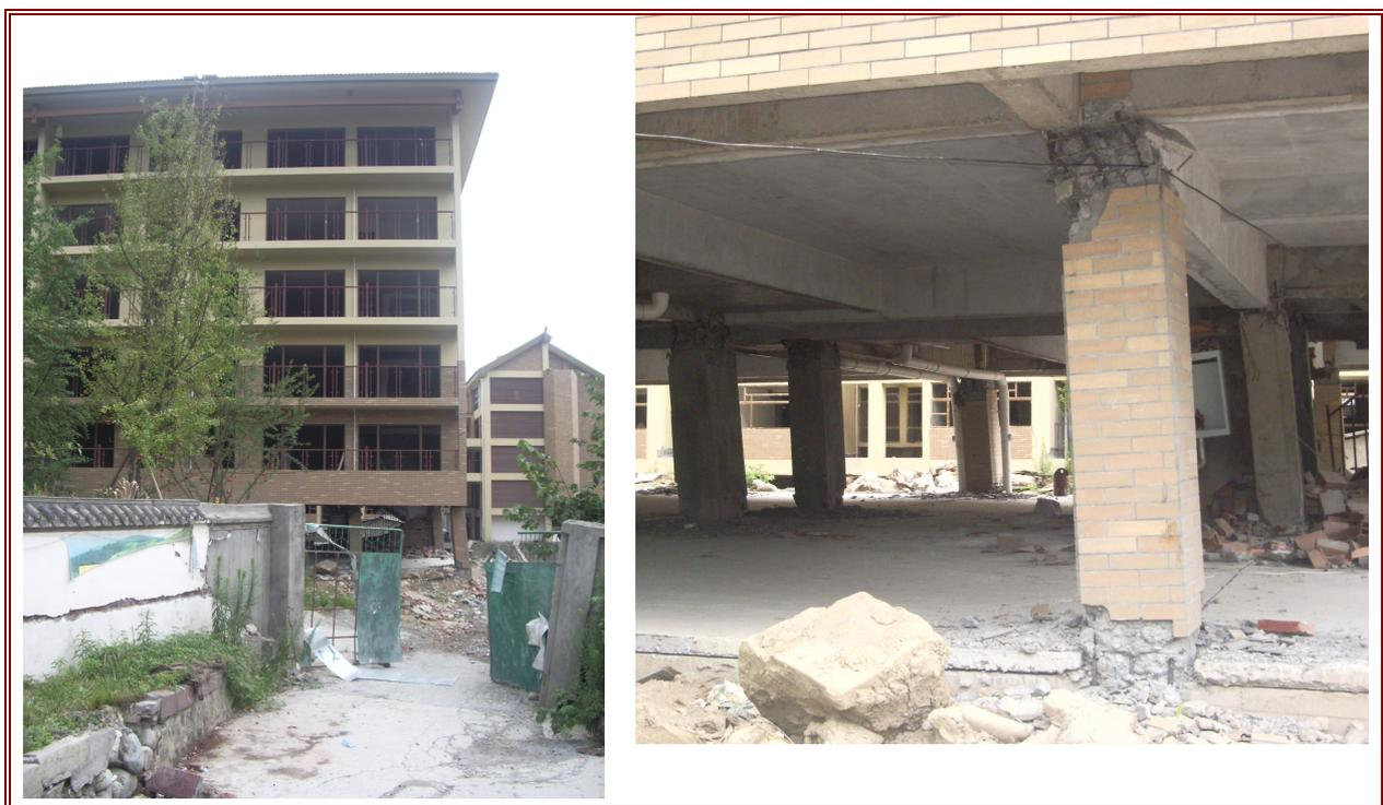
**Figure 3.1 Six-storey RC MRF in Yazhouyan housing development, Dujiangyan that is exhibiting a soft-storey failure mechanism at ground storey (detail of ground floor columns, right).**
