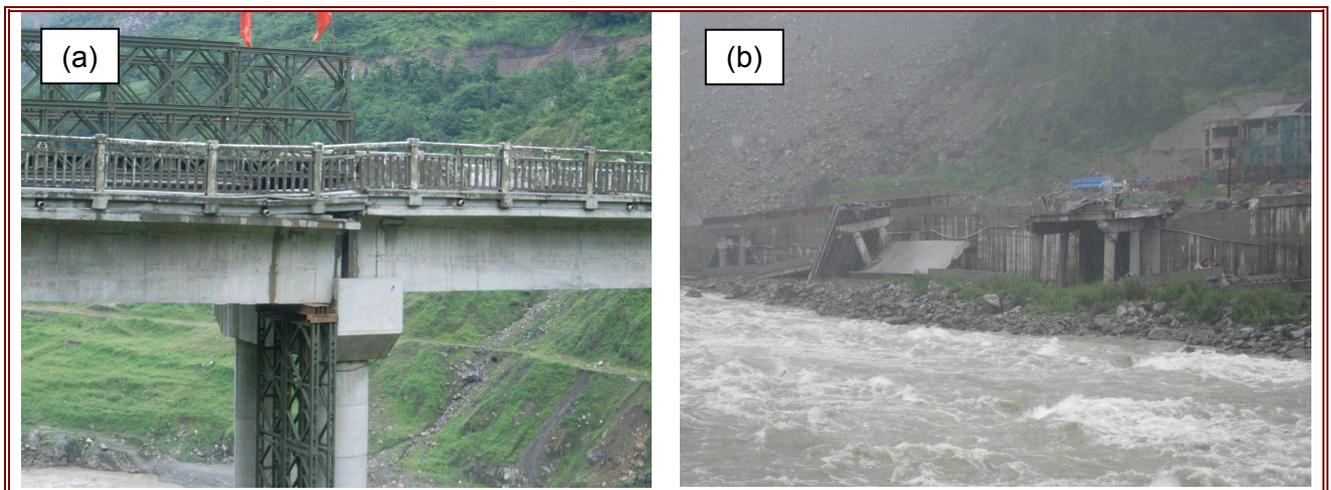
**Figure 5.1 Damaged bridges (a) Longitudinal displacement of simply supported beam at Shoujiang Bridge (b) Collapsed bridge viaducts along Mingjiang River in Ying Xiu Town.**
