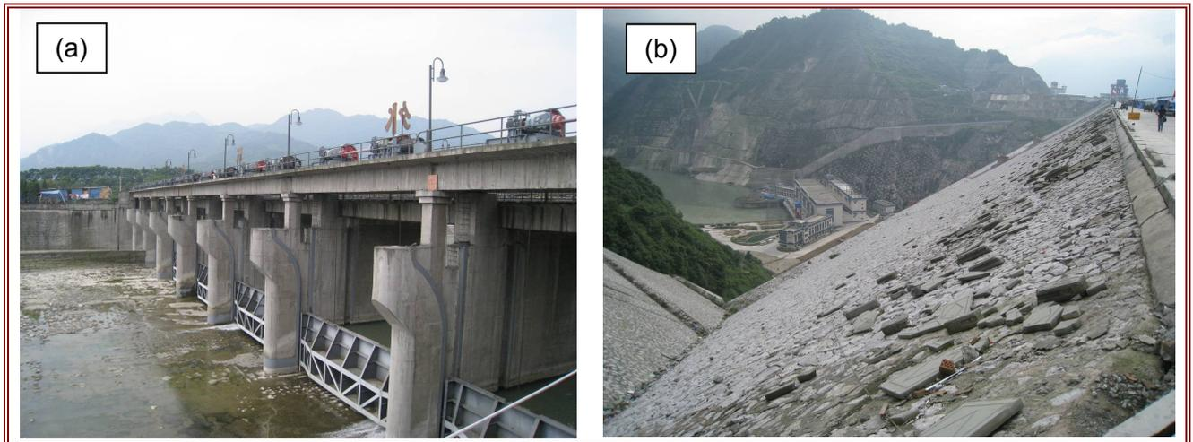
**Figure 5.4 Damage to Dams (a) View of dam at Dujiangyan Irrigation Project Fish Mouth where the beam that supported the dam gates experienced a 100mm lateral displacement in the downstream direction, and b) View of downstream side of Zipingpu Dam where cracking, slight bulging and differential settlement was visible at the crest (the loose slabs visible on the surface are from the collapse of a light-weight pedestrian footpath barrier along the crest of the dam).**
