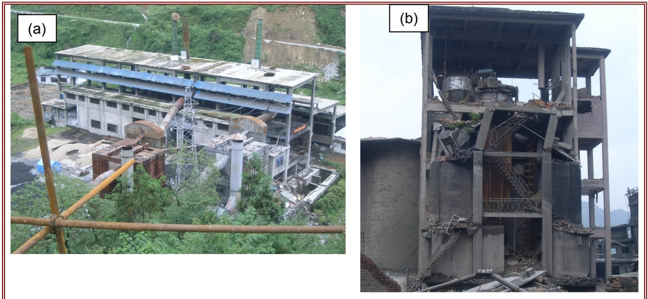
**Figure 4.3 Damaged cement factories in (a) Ying Xiu and (b) Xiao Yu Dong.**
