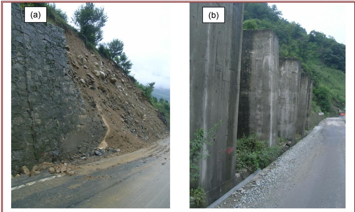
**Figure 2.2 (a) Collapsed section of stone gravity retaining wall near Ying Xiu (b) Displaced section of RC bored pile retaining wall stabilizing a pre-existing landslide to protect the road, near Ying Xu.**
