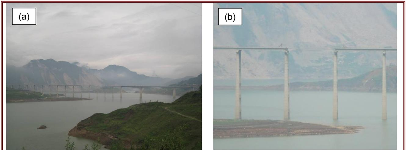
**Figure 5.2 Damaged bridges (a) shows Minjiang Bridge crossing the Zipingpu reservoir where one span is unseated. (b) view of missing span.**
