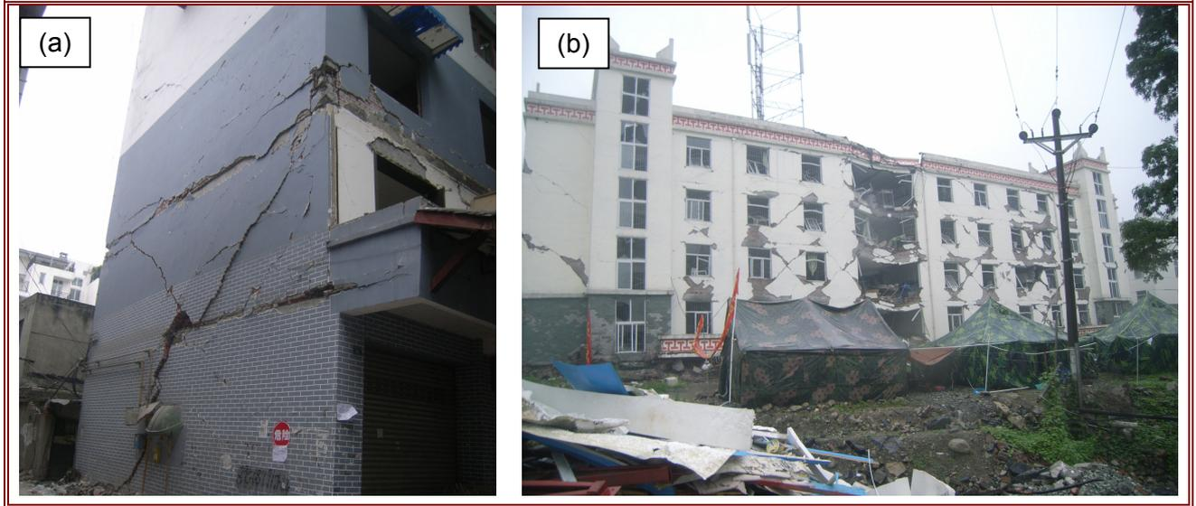
**Figure 4.2 (a) 5-storey confined masonry building in Dujiangyan with shear cracks on bearing walls, (b) 5-storey masonry school building in Ying Xiu partially collapsed.**
