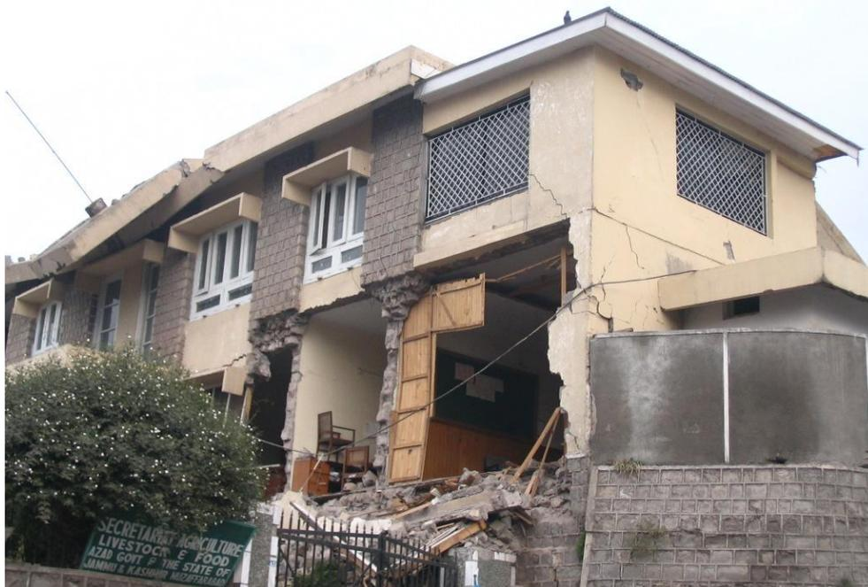
**Figure 3.39: Collapsed wall sections of the concrete block URM, 3-storey building of the AJK Secretariat of Agriculture, Livestock and Food. Collapsed RC slab roof, extensive damage**
