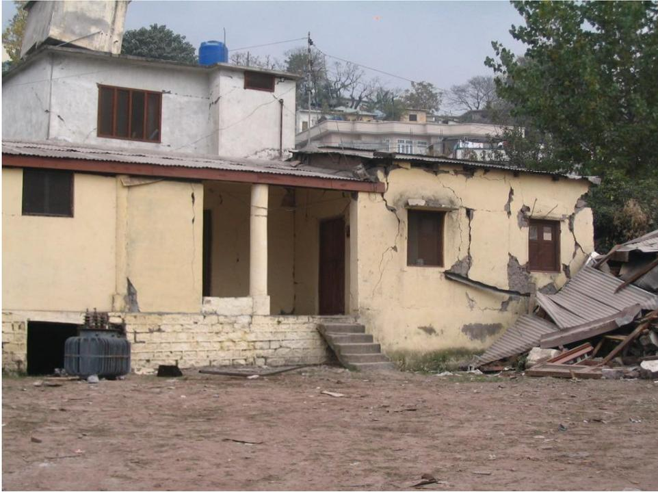
**Figure 3.23: Shear cracks through the concrete block masonry wall of a residential building, moderate damage, Muzaffarbad**
