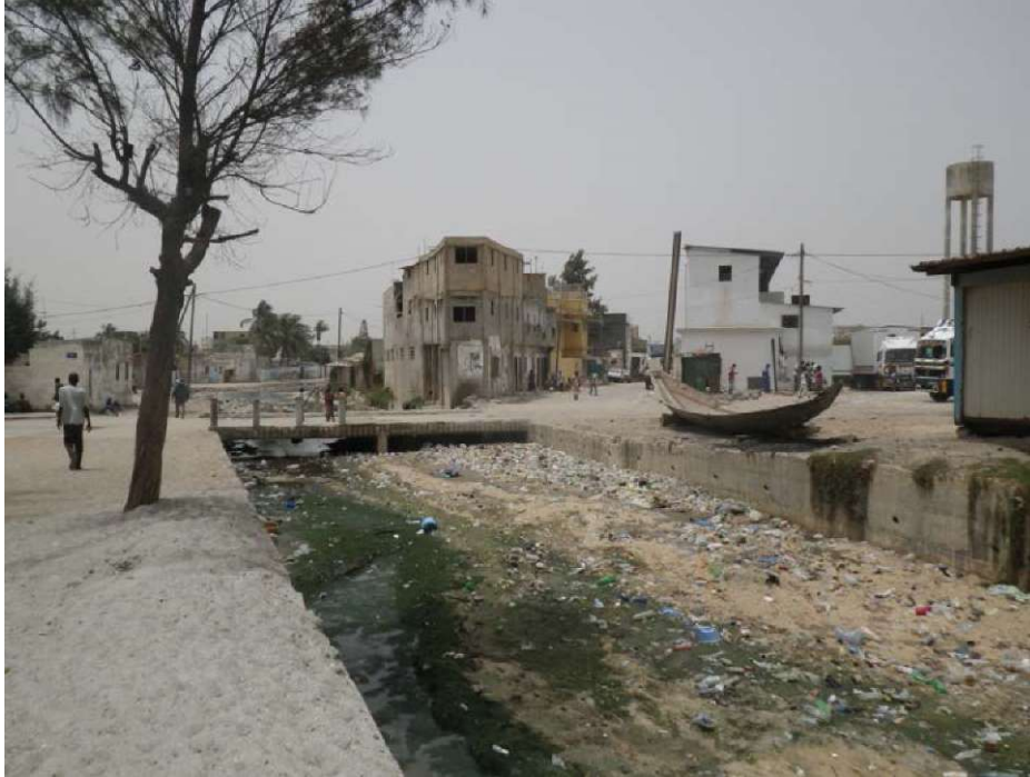
Photo 5: Drainage canal in Rufisque, cluttered with deposits (sand, refuse, waste water)
