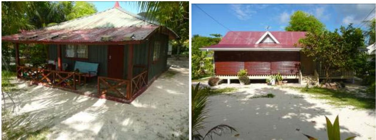
Figure 47 : Absence of protection and basement at same elevation than ground level in recent construction. On the right the recent house was build on an elevated basement.
