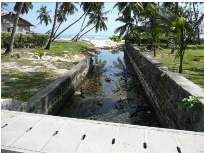
Figure 43 : channel draining a wetland in Silhouette island obstructed by reconstruction of a new beach at the outlet under the effect of South East monsoon (photo R. Guillande).
