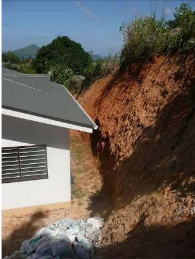
Figure 60: typical construction not respecting distance to slope and base and stability angle of slope (photo R.Guillande).
