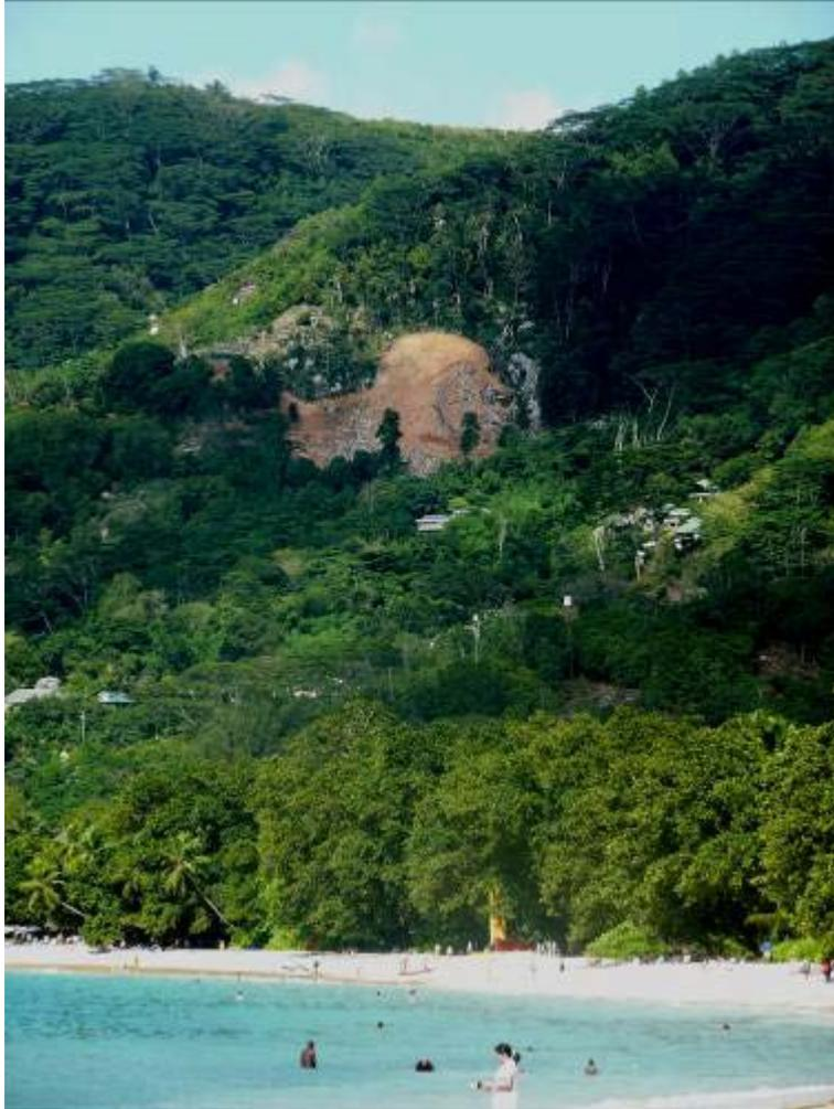
Figure 55 : landslide above Beau Vallon bay caused by destabilisation during earthwork for a new construction (photo R. GUILLANDE).
