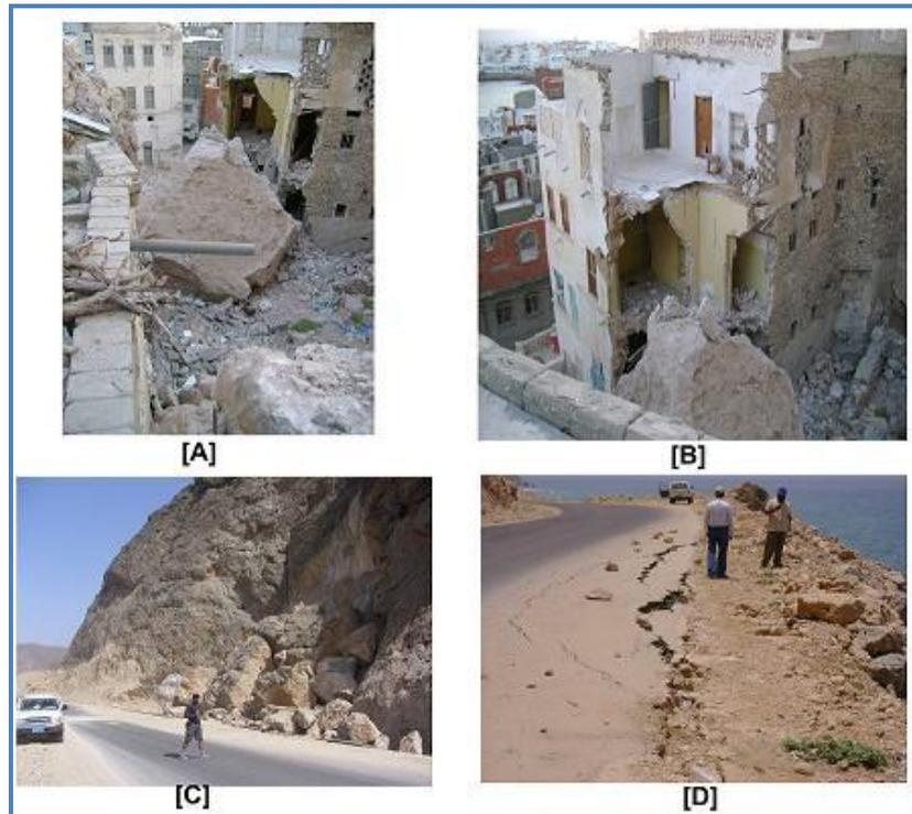
Figure 4-7: A, B: Rockfall destroyed houses in Al-Mukalla city. C Rockslide occurred along the road between Al-Ghayada and Howf. D Cracks developed on the road
