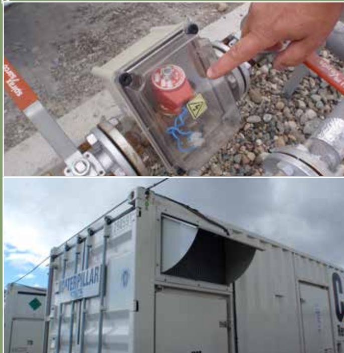
Adaptations to protect GenSet equipment in Bariloche, Argentina, from repeated airborne ash exposure following 2011-2012 eruption of Cordon Caulle volcano, Chile. Top: sealed fuel valve. Bottom: hood to protect air intake.
