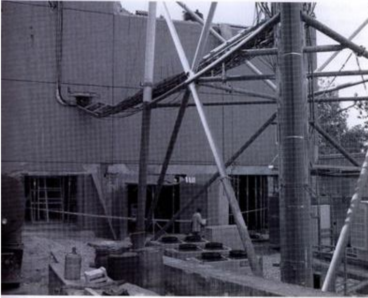
Figure 19 Damaged Cable Tray from Tower to data Center at Haiti Cellular Phone Company
