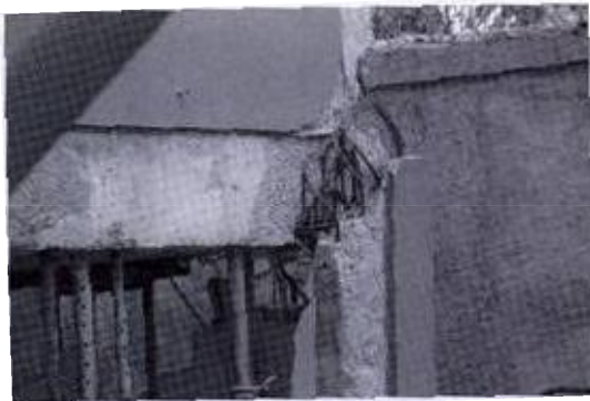
Figure 18 Failure of Beam-Column Joint Close to Cable Tray Attachment to Building
