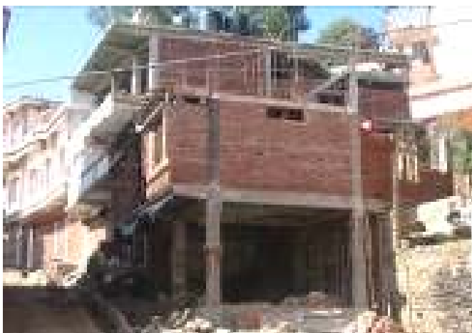
Figure 35: A new building with incorporation of earthquake-resistant elements learnt from MDRIP training
